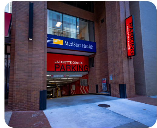
Lafayette Centre 21st Street garage entrance
