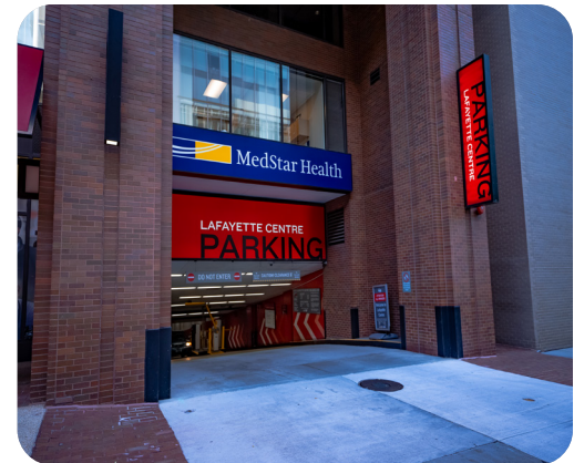
Lafayette Centre 21st Street garage entrance
