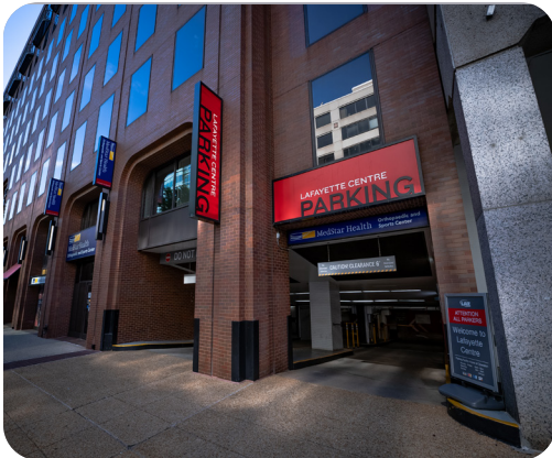
Parking garage entrance from 20th Street
